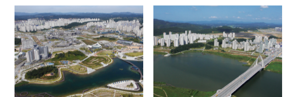
Construction of Sejong Metropolitan Autonomous City (MAC)
