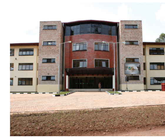
Facility Aid (ICT Building in University of Rwanda)
