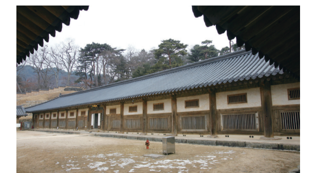
1 Haeinsa Temple Janggyeong Panjeon (1995) Hapcheon, Gyeongsangnam-do; photo of Janggyeong Panjeon This building, as the oldest annex of Haeinsa Temple, was designed for preserving the Tripitaka Koreana woodblocks in a way which takes into account environmental conditions like temperature, humidity, and ventilation.
