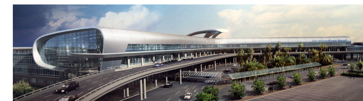
Jeju International Airport
