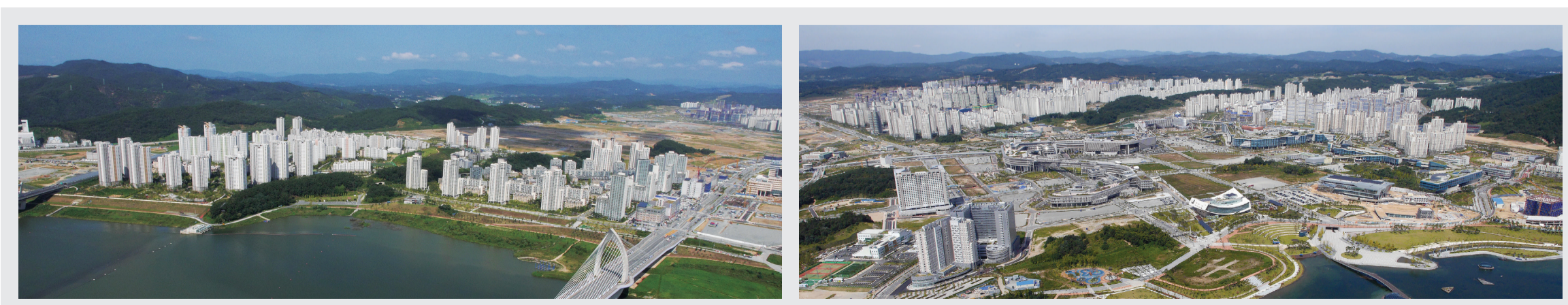
Construction Sites of Sejong Special Autonomous City
