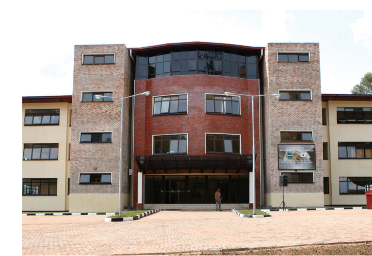
Facility Aid (ICT Building in University of Rwanda)
