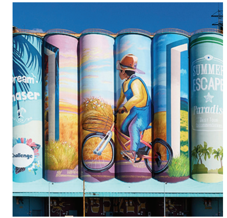
Silos to Store Imported Grains
