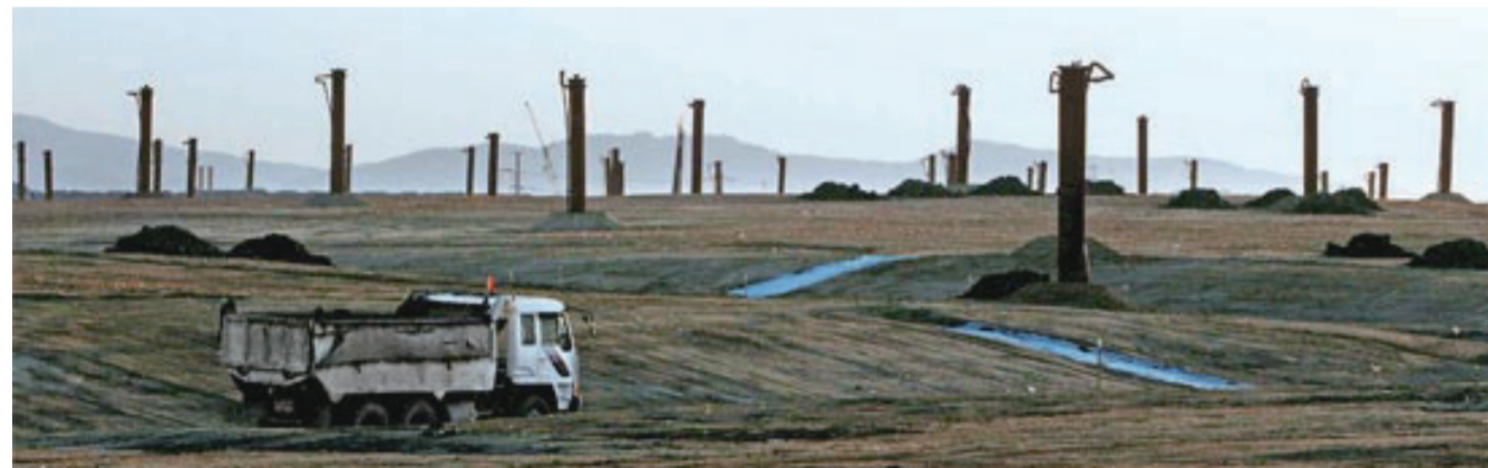
Soil covering at the Metropolitan Landfill site. The poles are built to capture methane gas for use in generating electricity
